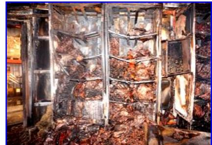
These units are used as backup power for computer server farms, valued at over \$1,000,000 each. One was damaged by fire and another suffered heavy smoke damage. (Above photo by Franklin Fire Dept. All other photos this page by Chuck Liedtke)
